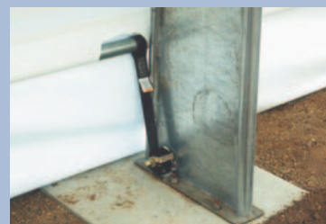
BOTTOM TRUSS CONNECTION
